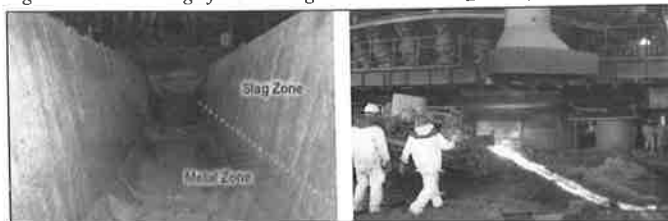
Fig. 4: Application of trough castable
