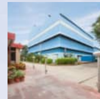
Almatix Alumina Private Ltd., Falta, India
