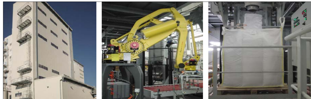
Fig. 2 New crushing centre at Almatris Ludwigshafen plant
